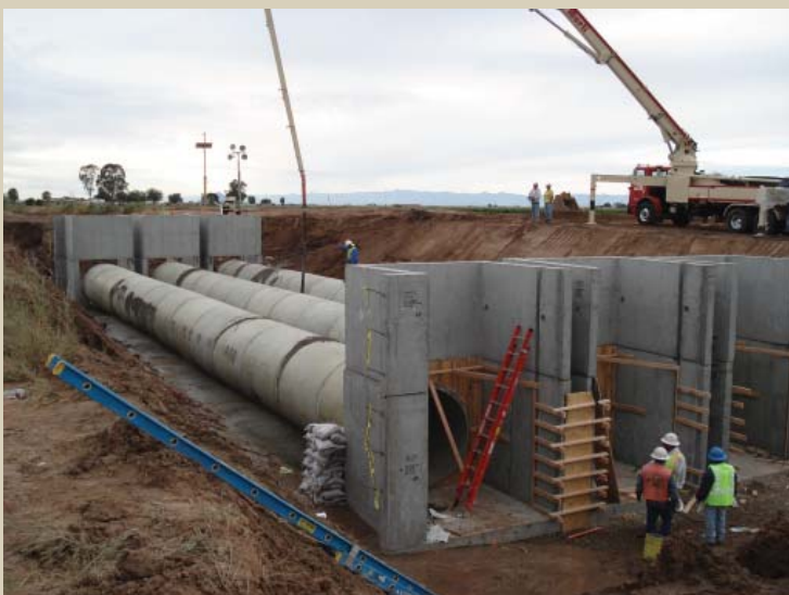
(Left) IID water construction crews build and (right) pour concrete slurry to encase three 72-inch pipes that will move water along the Westside Main Canal as it is routed under the road to accommodate the Highway 111/78 Brawley bypass.
