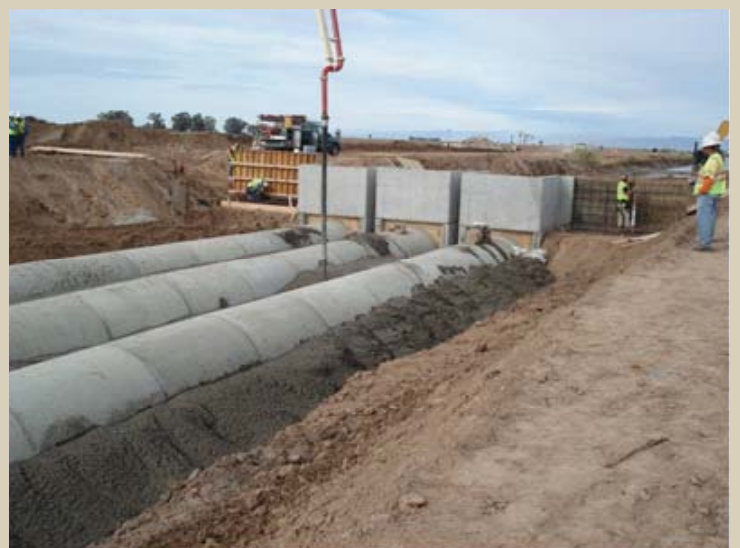
(Left) IID water construction crews build and (right) pour concrete slurry to encase three 72-inch pipes that will move water along the Westside Main Canal as it is routed under the road to accommodate the Highway 111/78 Brawley bypass.
