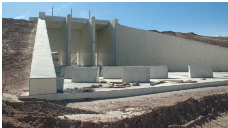
One of the inlet structures at the Drop 2 reservoir.
