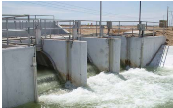
Above: The offline storage reservoir's inlet structure with its gates open. Below: The reservoir was filled for the first time in late August.
